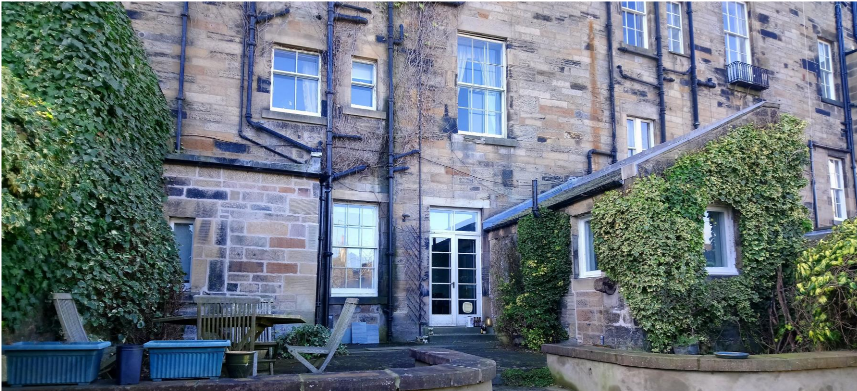
View 1 External view from lower garden
