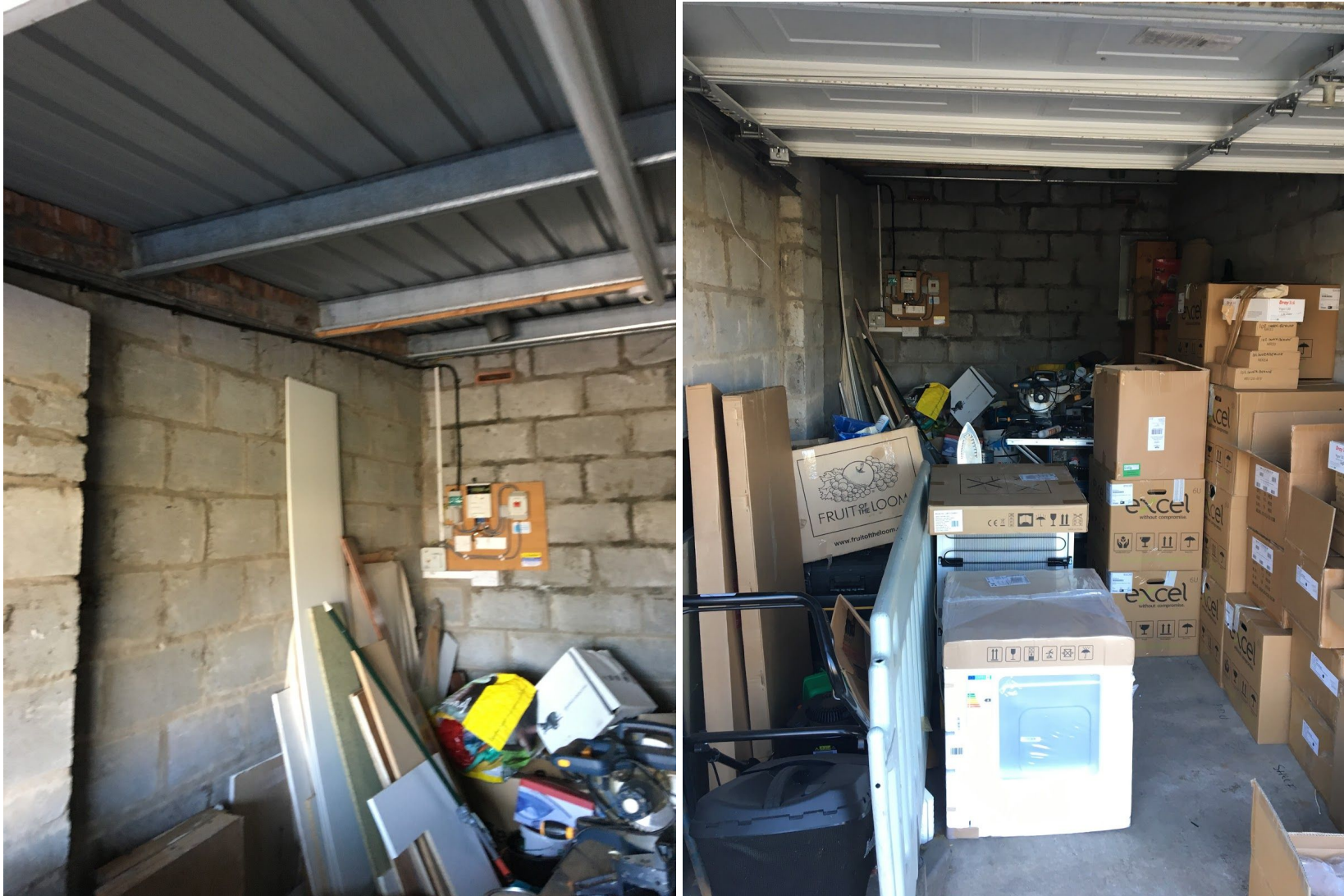
Internal photos of existing garages
