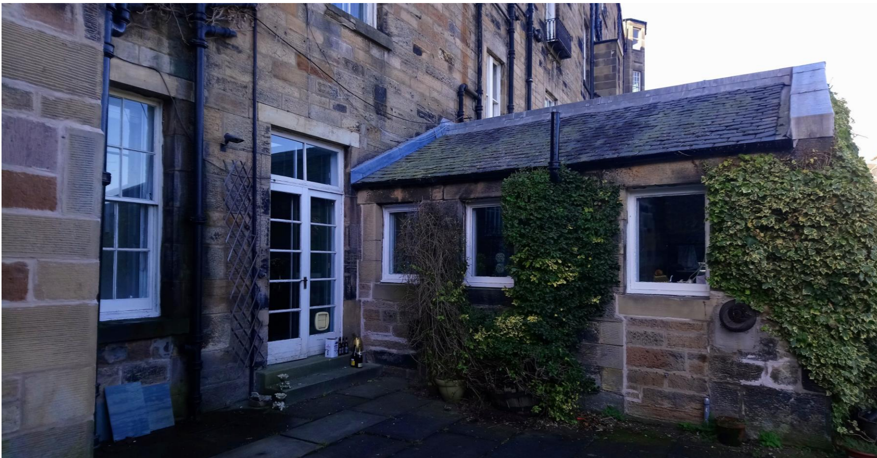
View 2 External view from terrace.
