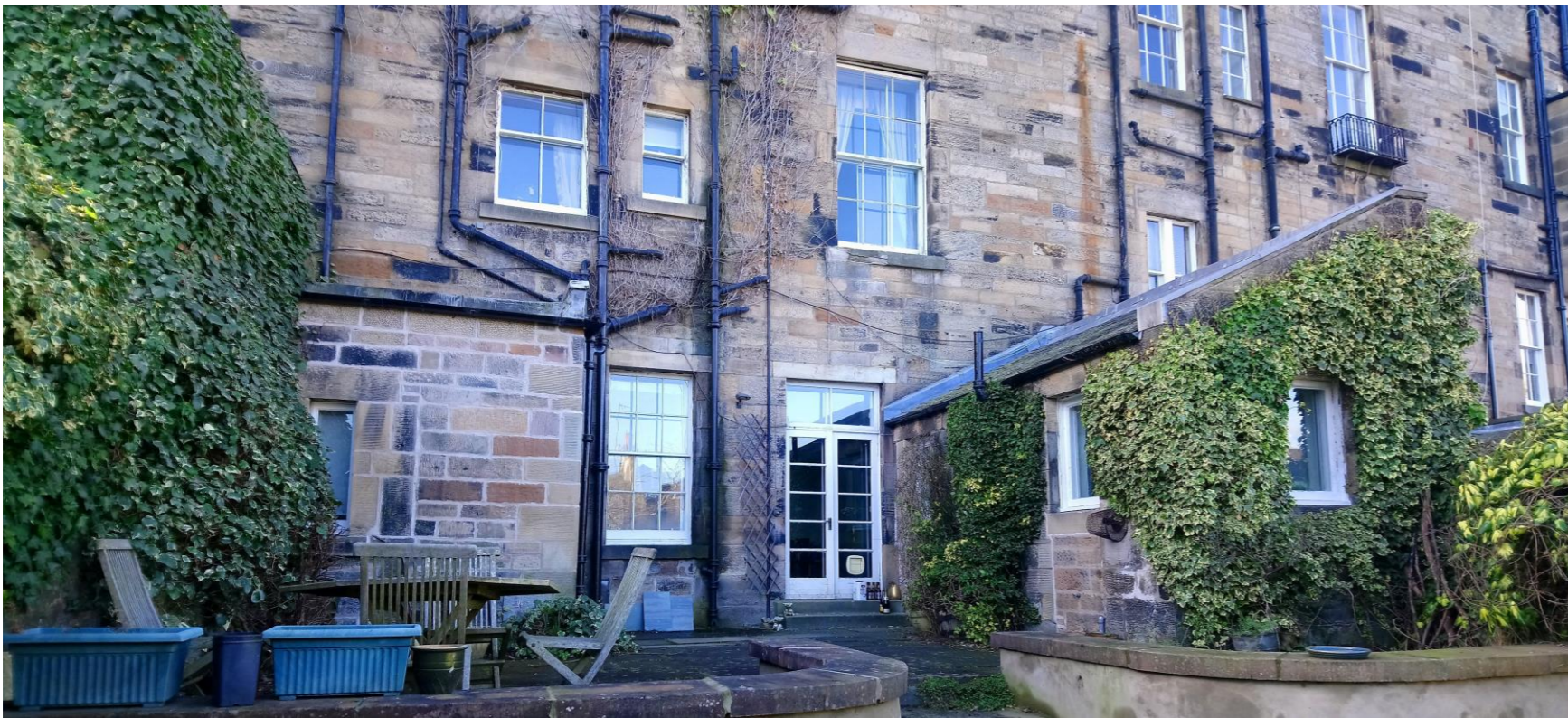
View 1 External view from lower garden
