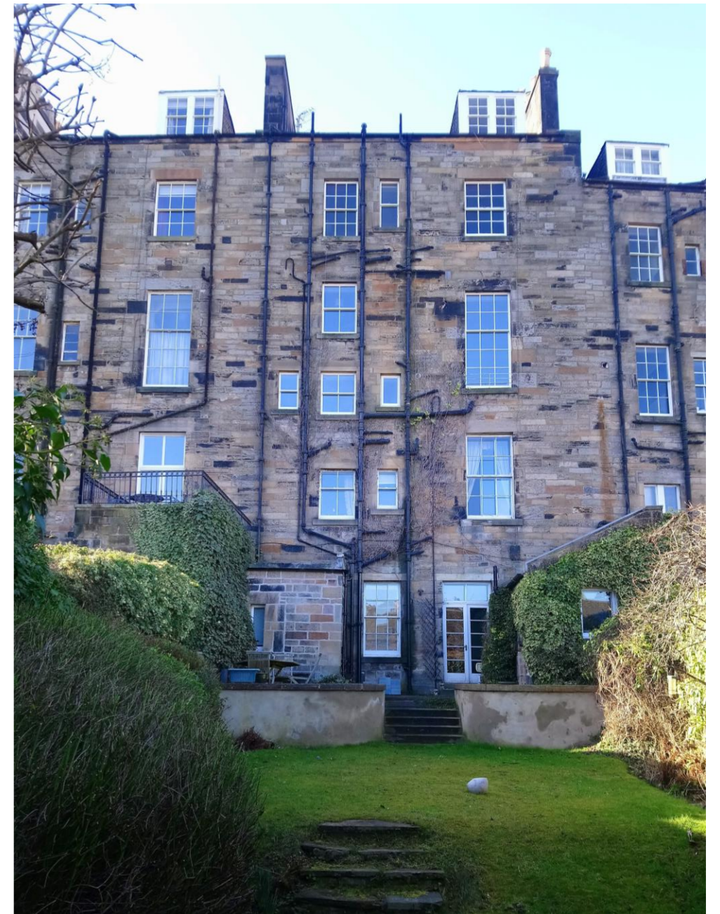
View 3 Full rear elevation from garden
