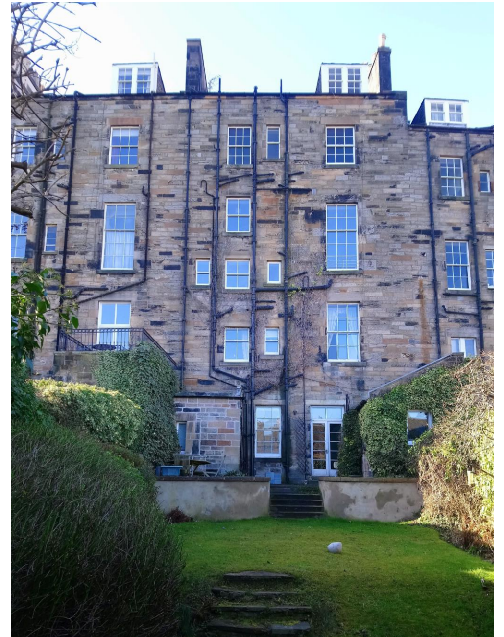
View 3 Full rear elevation from garden
